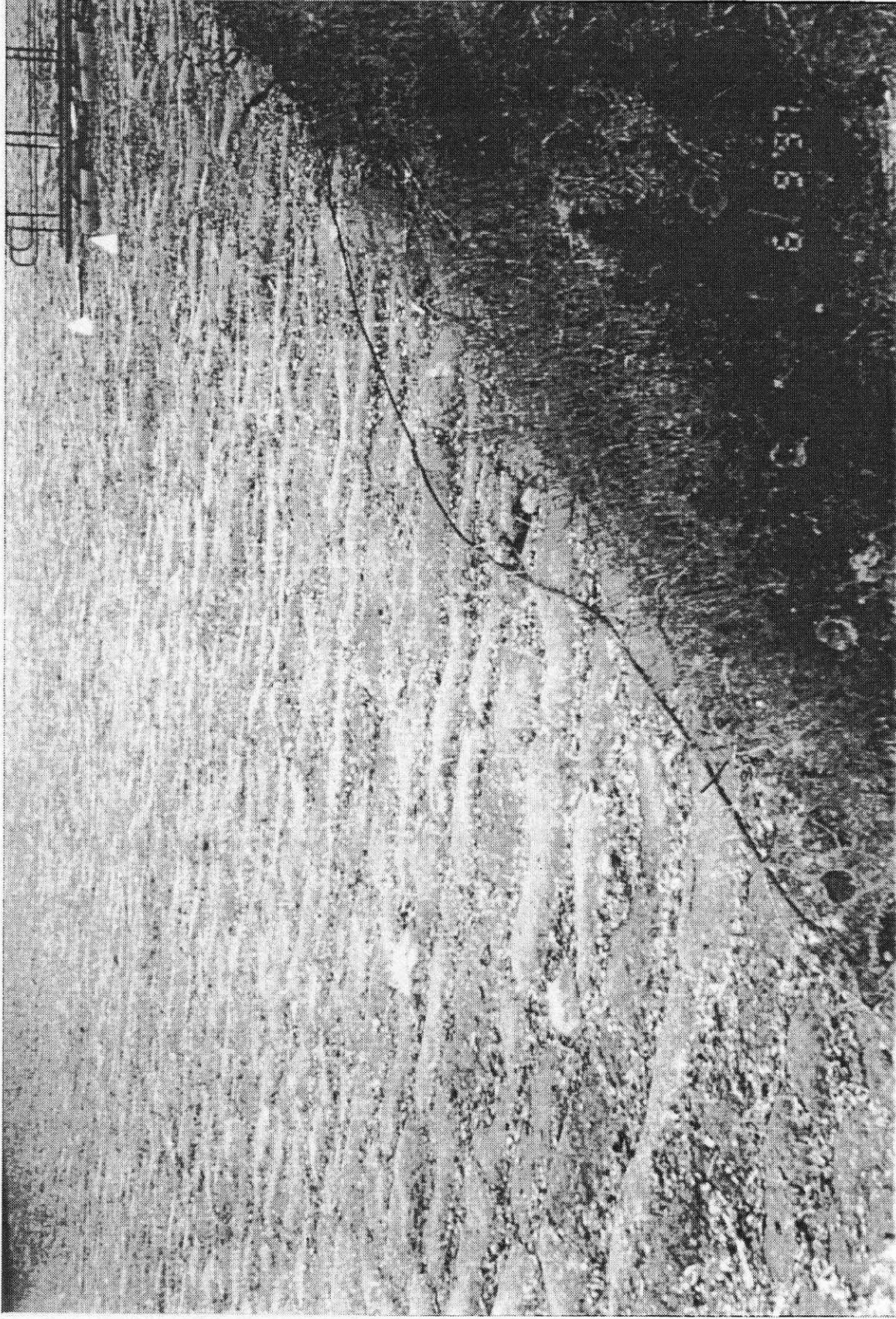
Figure 5.3.1 Depoist of chemical wastes in a former opencast mine at Wolfen, Germany. The surface is covered with biological filters protecting against H_2S emissions
