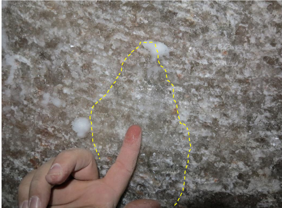
Fig. 1. (A) Brine inflow rates measured in different (as indicated by different colors) unheated boreholes 37 and (B) patch-wise brine wetting and weeping observed on tunnel surfaces (courtesy of Doug Weaver, Los Alamos National Lab) at the Waste Isolation Pilot Plant. In B, yellow dash line is added for visual guide.
