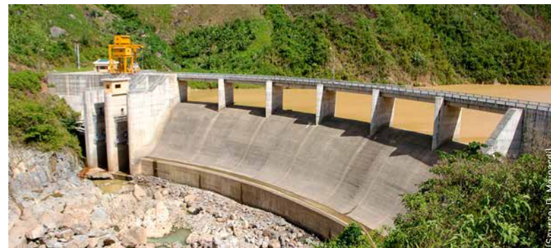
Za Hung dam used for hydroelectric power in a tributary of the Vu Gia river in the Dong Giang district, Quang Nam province.
