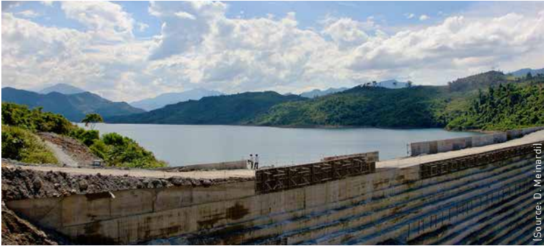
Final operations on the dam Song Tranh 2 in 2011 in the district of Bac Tra My, Quang Nam province.
