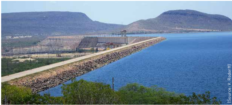
The dam wall of the Itaparica Reservoir with six hydro-electric turbines, each with a capacity of 250 megawatts.
