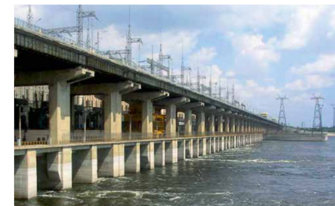
Fig. 65: Volga barrage at Volzhskaya → Photo: KIT/IMB
