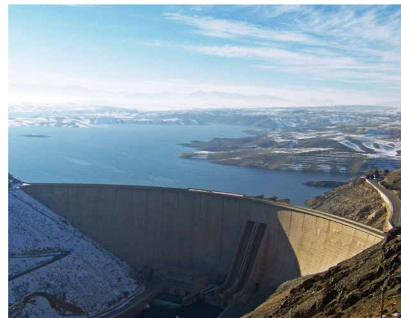
Fig. 53: Chadegan Dam on the Zayandeh Rud. → Photo: p2m berlin GmbH
