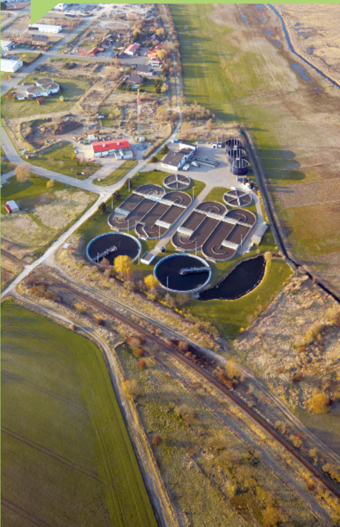
Fig. 14: The interactions between the natural and technological compartments are of prominent importance in Urban Water Resources Management.
