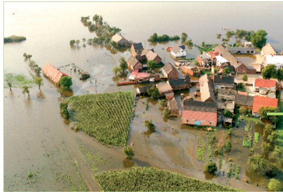
Fig. 18: Floods threaten settlements and infrastructure; as recently seen along the Elbe in June 2013.
