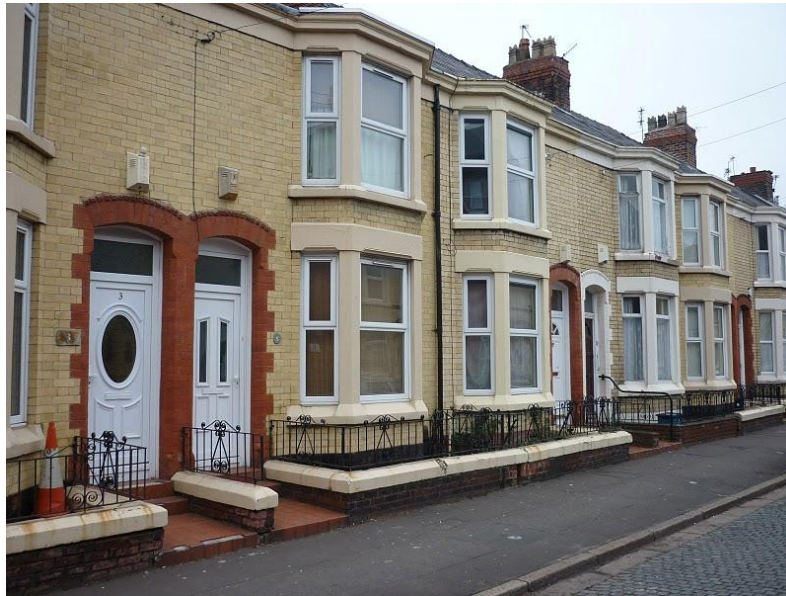
Figure 16. Refurbished housing in Kensington.
