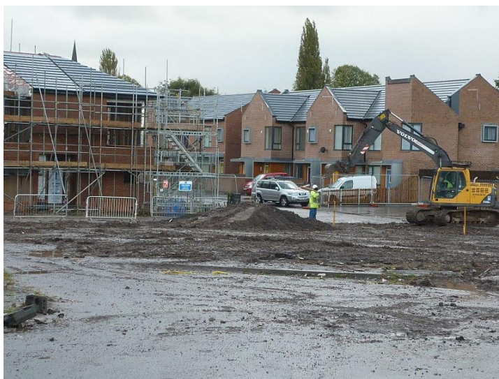
Figure 9. Replacement housing being built on a slum clearance site at Fiveways, Rock Ferry.
