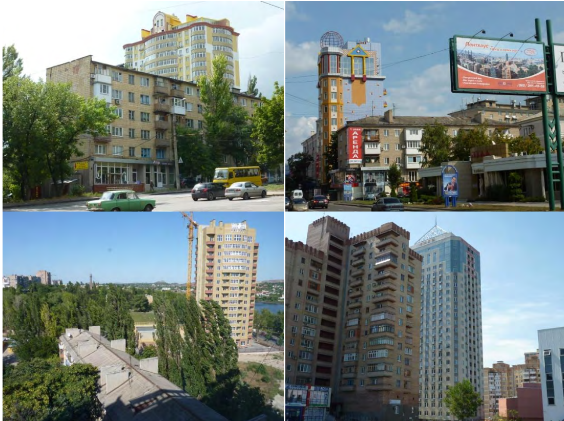
Figures 84-87 Newly-built blocks of flats, central Donetsk, 2009
