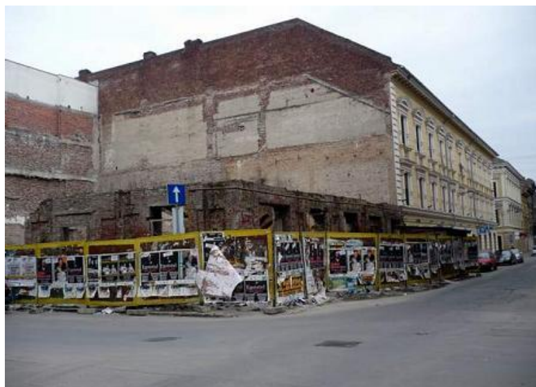
Figure 34 – Demolished building into the historical centre
