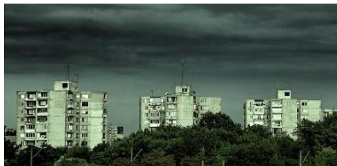
Figure 7 – 10 levels blocks into the summer storm
