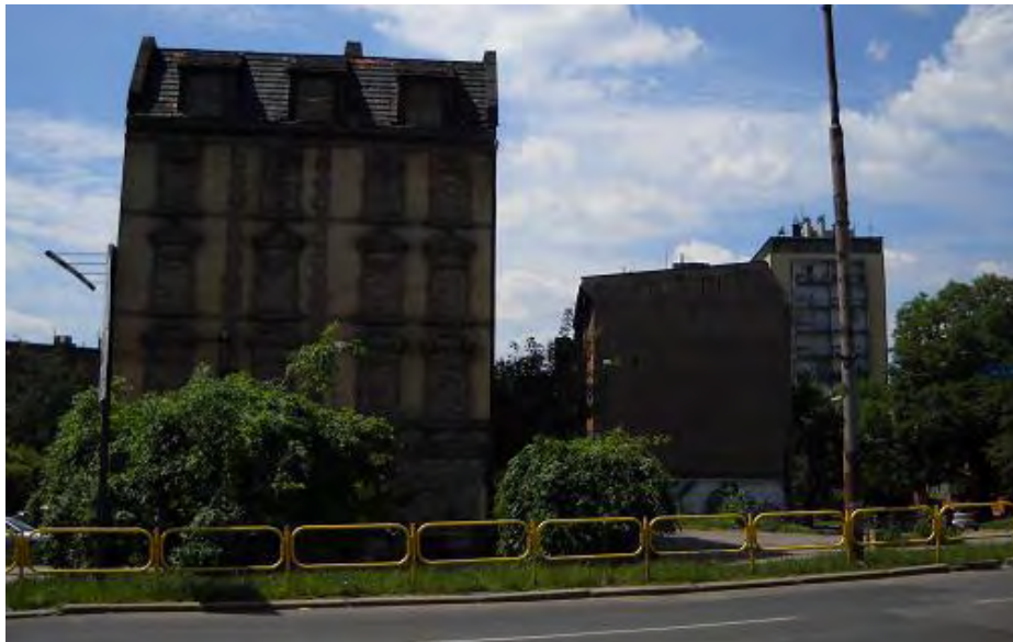
Figure 7. Tilting of buildings as an effect of mining damages in Bytom
