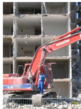
Figure 3.4.7: Demolition of housing
