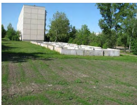
Figures 3.6.3: Post-demolition brownfield
