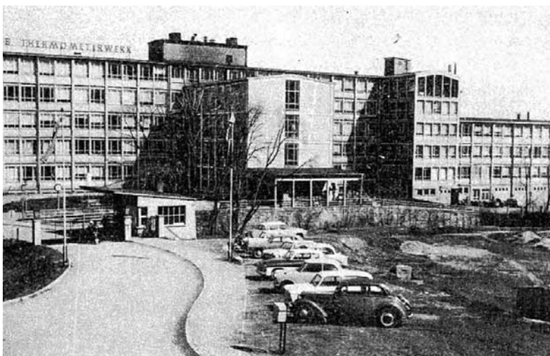
Former Nationally-Owned (VEB) Thermometer Factory, 1960
